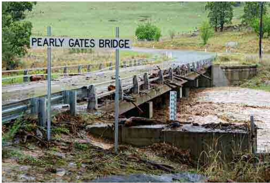
Debris at Pearly Gates Bridge, Peel River upstream of Nundle, 2010 flood Source: Kerrie Fearby
