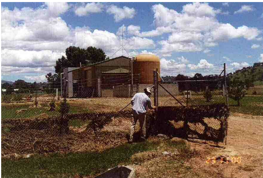
Debris line at water treatment plant, Hall Street, Nundle, after 2000 flood
