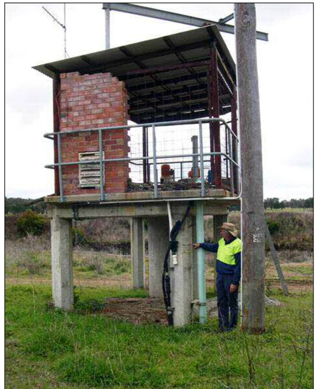
Nundle Pump Station, showing the level of historical floods. The November 2000 flood reached to the middle railing.
