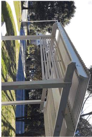
Shelter structures; aluminium structures with skillion roofs
