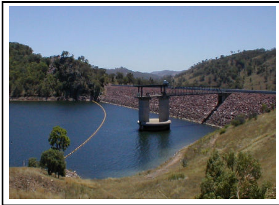
Figure 3.13 Chaffey Dam showing spillway and rock wall
