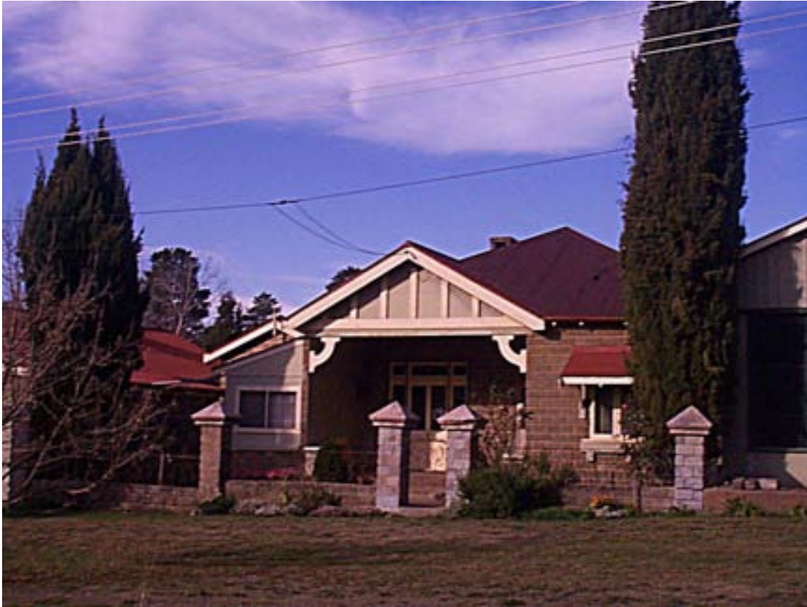
The interesting aspect of this inter-war bungalow from Woolbrook is the material from which it is built. The concrete blocks are a feature of the town, and are indeed unusual and rare as a building material. A number of buildings in Woolbrook in the 1920s were constructed with this material.
