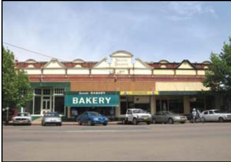
Figure 48: Treloar's Buildings, Barraba, 2006. Photograph courtesy EJE Group.
