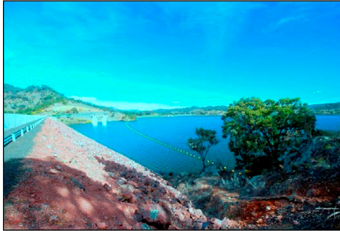
The Chaffey Dam wall
