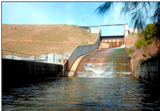
The spillway at Dungowan Dam
