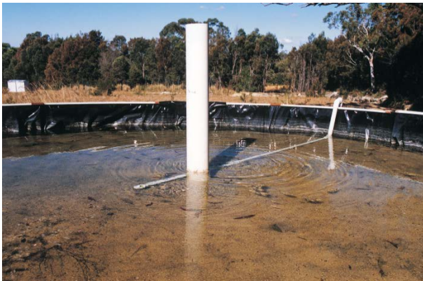
Figure 15. Slow sand filtration can control some plant pathogens at flow rates between 100 and 300 L/m 2 /h.
