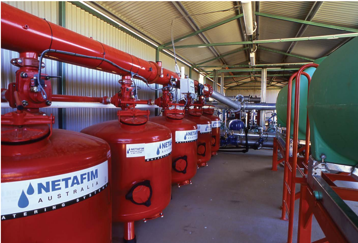
Figure 21. Media filters are effective for removal of organic material and fine sediments.
