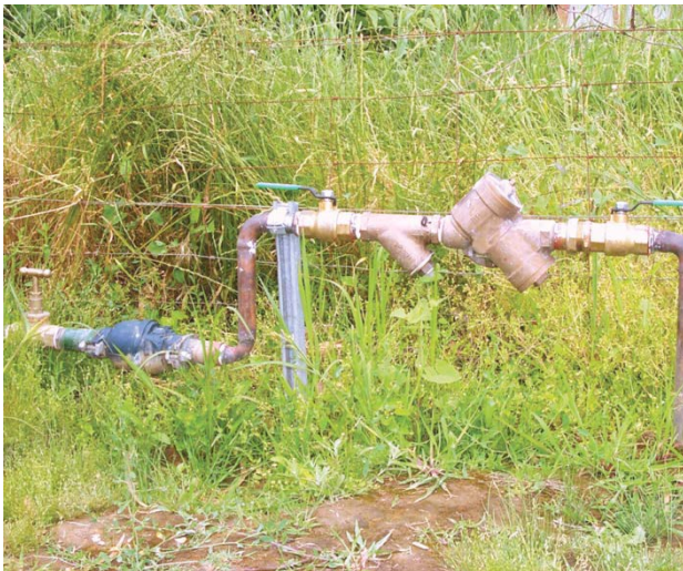
Figure 17. When using chemical solutions in an irrigation system on town water, a suitable backflow device is required to stop reversed flow to the water service.
