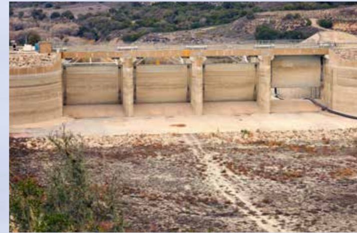
Santa Barbara, California, USA - January 1, 2016: Falling water levels at Lake Cachuma due to severe California drought leave the locks at Bradbury Dam high and dry.
